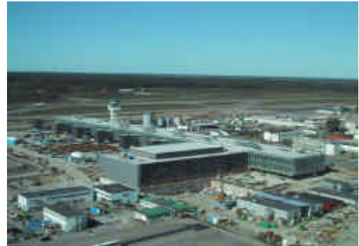
Photo of the new Pier F
